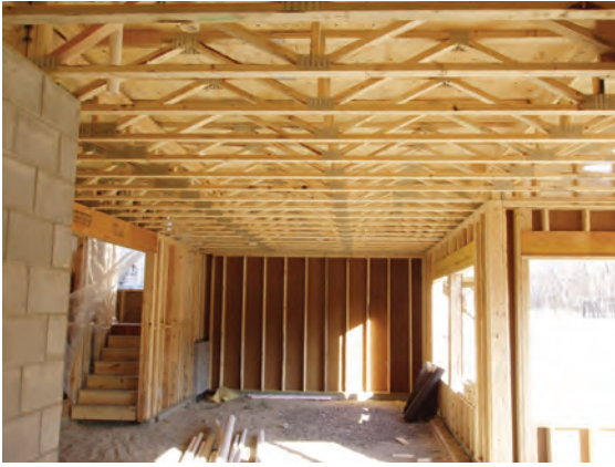
FIGURE 6-4 Open-web floor trusses
