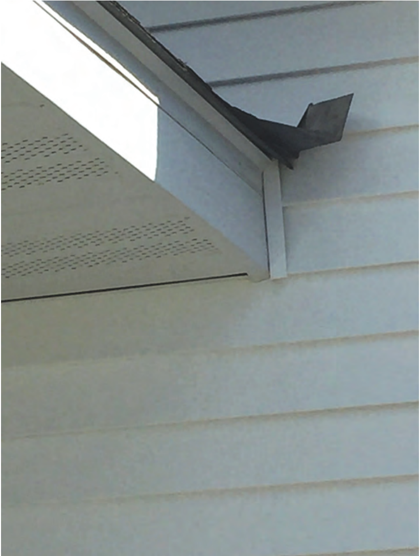
FIGURE 7-13 Kick-out flashing for asphalt shingles
