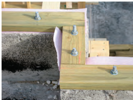
FIGURE 5-12 Anchor bolts in a wall offset
