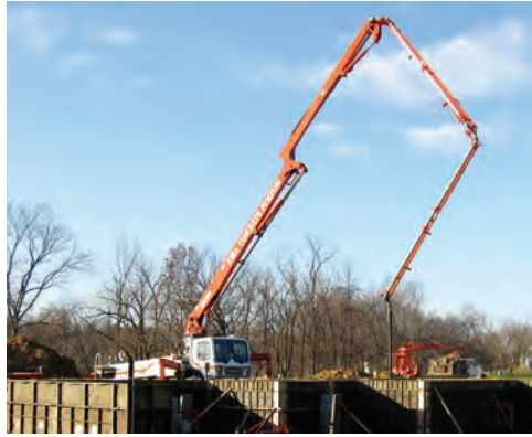
FIGURE 5-2 Pump to place concrete for the basement of a single-family dwelling
