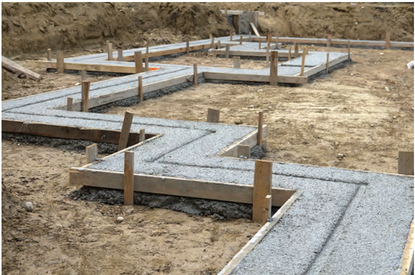
FIGURE 5-10 Concrete spread footing
