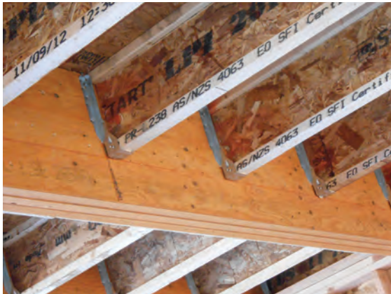
FIGURE 6-3 Engineered wood products: I-joists and LVL beam
