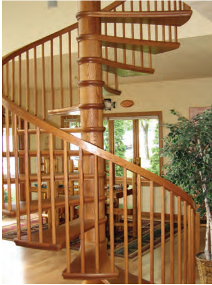
FIGURE 8-1 A spiral stairway is one type of stair permitted as a means of egress
