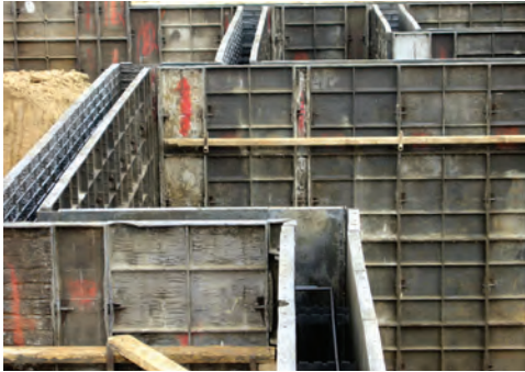
FIGURE 5-1 Concrete foundation forms for a single-family dwelling
