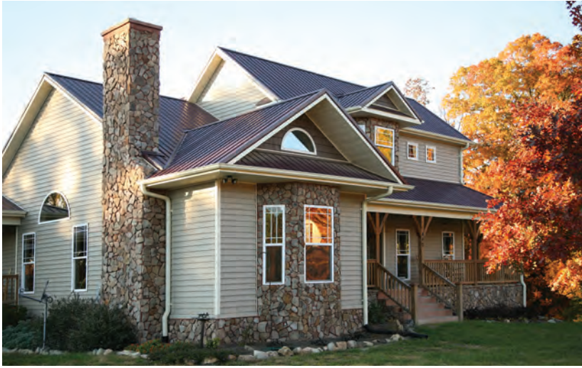
FIGURE 11-1 A masonry chimney is constructed of solid masonry units, hollow masonry units grouted solid, stone or concrete.
